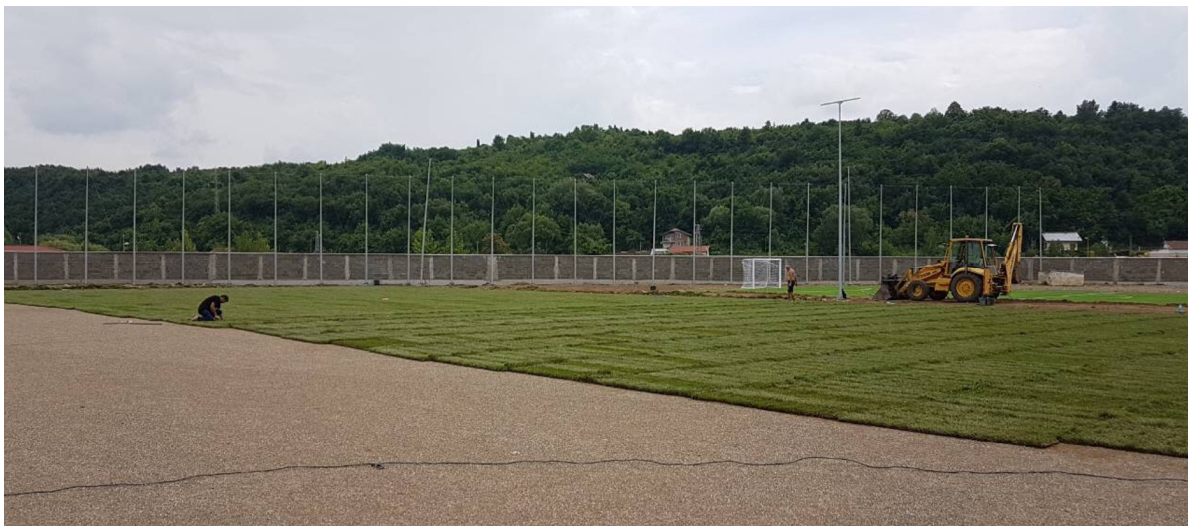
Stadium in Montana, work in progress
